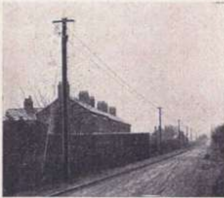
LOW-TENSION OVERHEAD LINE, WITH B. OF T. GUARDS.
